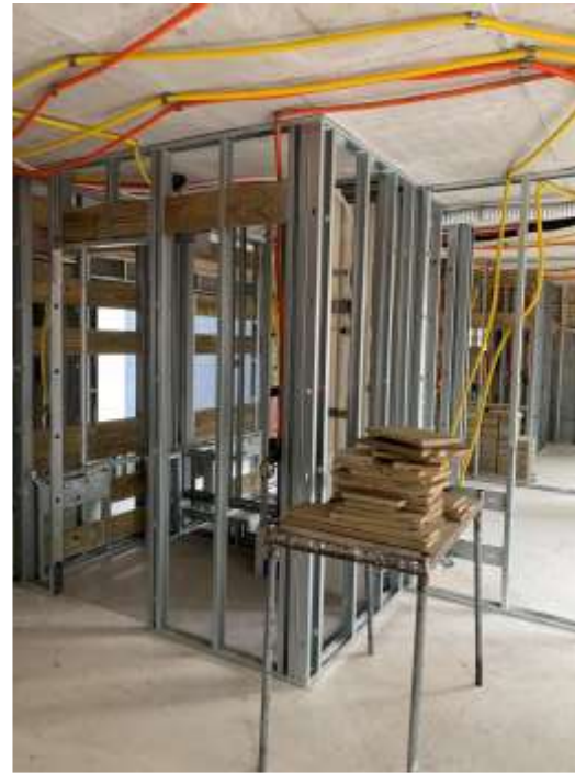
Ready to install electrical wiring
