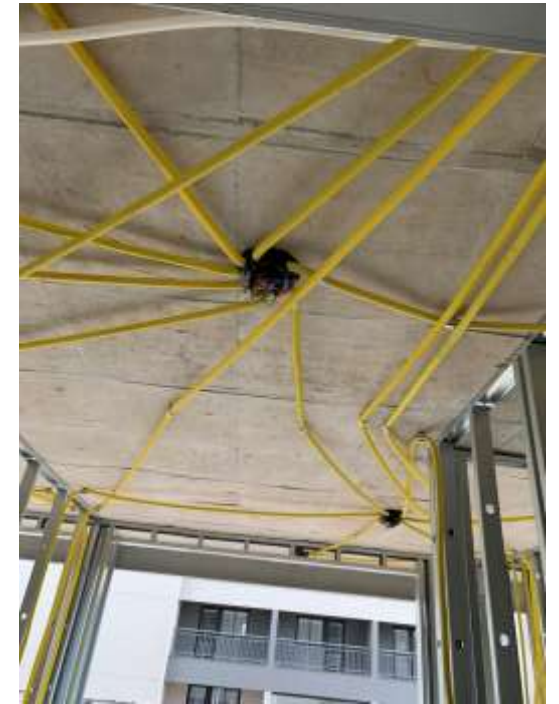
Ready to install electrical wiring
